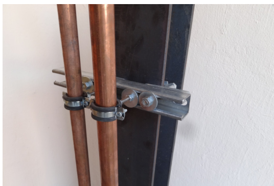
Simple pipe guidance on steel beams
