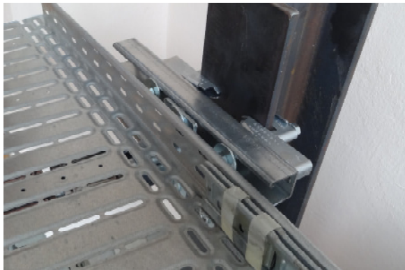
Quick fixture of a cable channel
