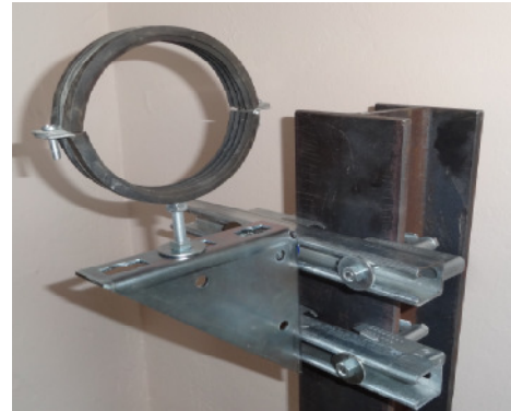
Installation of a bracket console
